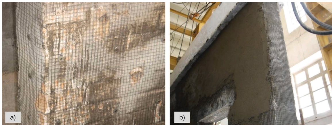
Fig. 1. – (a) Reinforced plaster application of wire mesh and (b) application of plaster [32].
